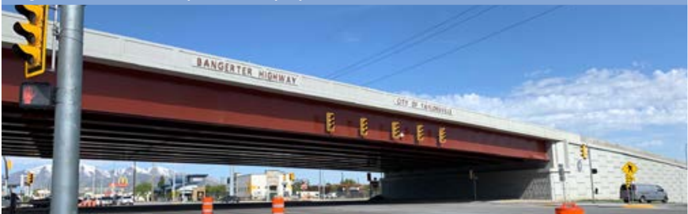
FIGURE 3.11 Existing structure that carries Bangerter Highway over 5400 South. Figure illustrates example of what proposed structures would resemble.
